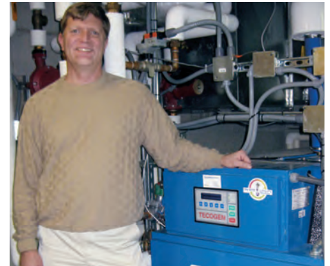
Paul Lund, Director of Facilities, stands next to CWV's new 75 kilowatt electrical cogeneration unit in The Village's Skilled Nursing Center.
